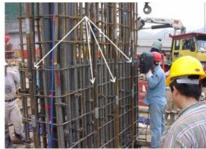
Tube-a-manchette Installation
