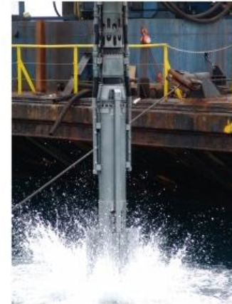
Offshore Vibro Compaction
