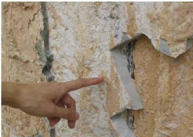
Grouting layer after completion
