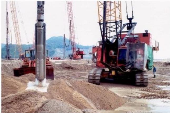
Land Based Vibro Compaction
